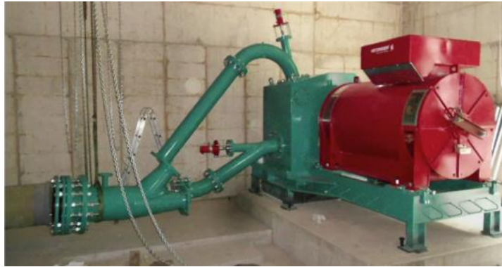
Fig. 2.7 Turbina Pelton [6]
